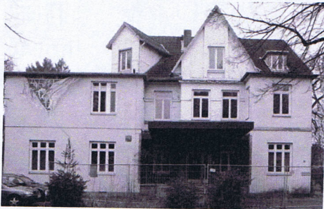
Manhagener Allee 56 Bestandsituation
