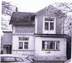
Manhagener Allee 54 Bestandsituation
